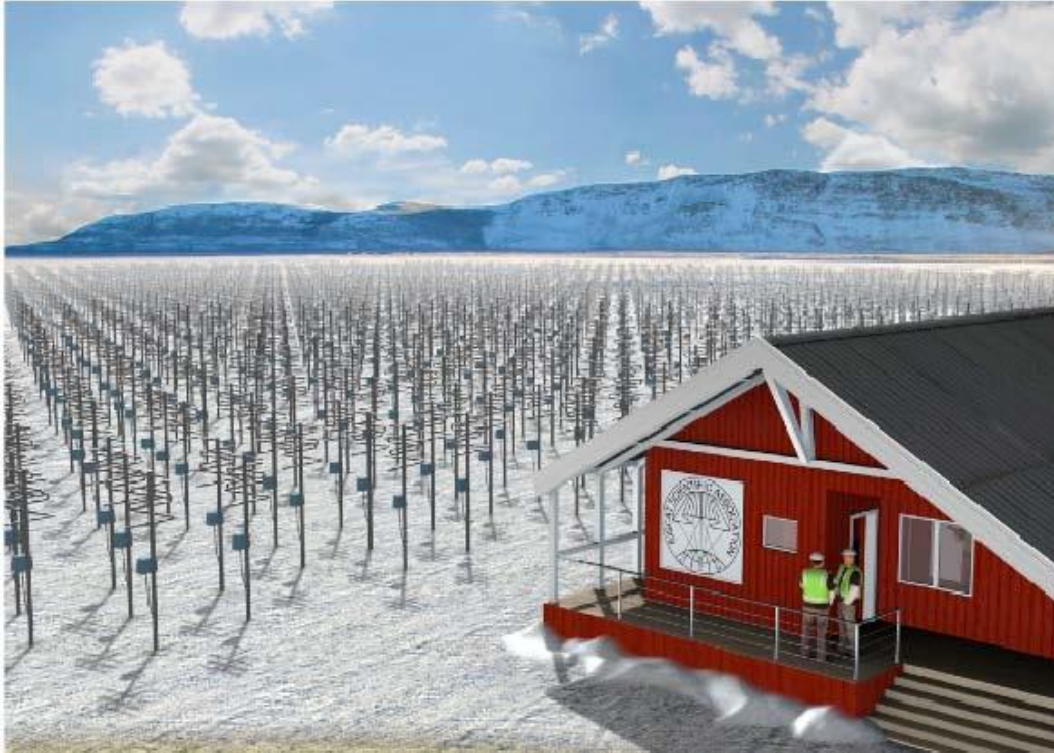
Figure 1: Artistic view of a phased-array transmitter for EISCAT_3D. Current plans include 32,000 phased array elements for the transmitter and 16,000 for the receiver sites.
